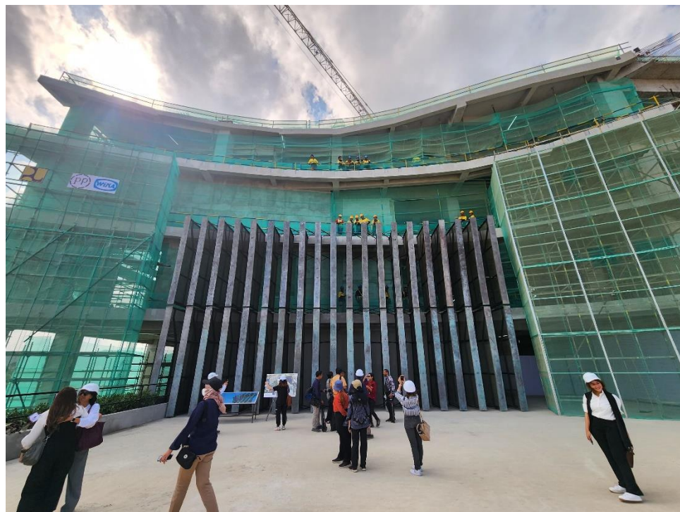
The front view of the State Palace is still under construction.
