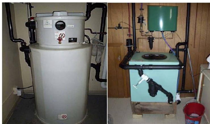
Gambar 21. Unit Brac Greywater Reuse System (kiri) dan iDus Controls' Conserve Pump system (kanan)
